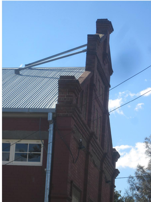
Figure 16. A closer view of parapet stays.
