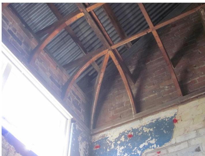
Figure 34. Ceiling joists of former Lodge Room, showing curved cornice brackets.
