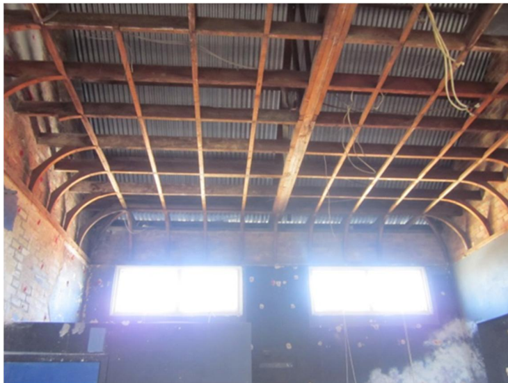
Figure 36. Ceiling joists of former South (supper room in eastern portion of building), showing curved cornice brackets.
