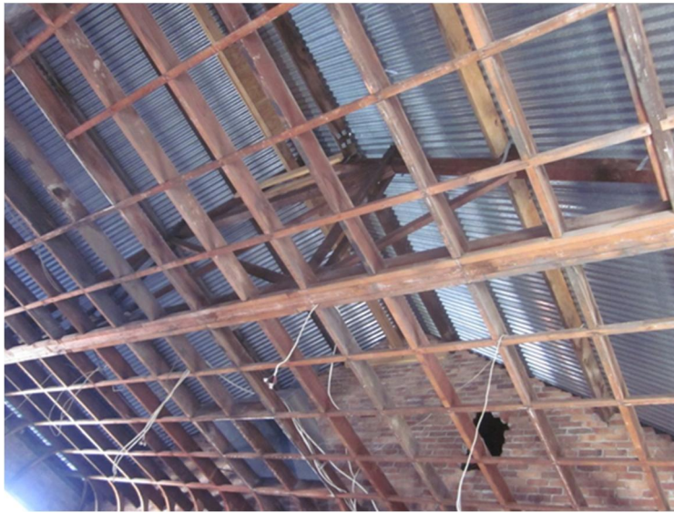
Figure 35. Ceiling joists of former Lodge Room, with roof truss visible beyond.
