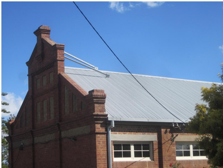
Figure 17. Facade parapet from Lakeview Street; note parapet stays.
