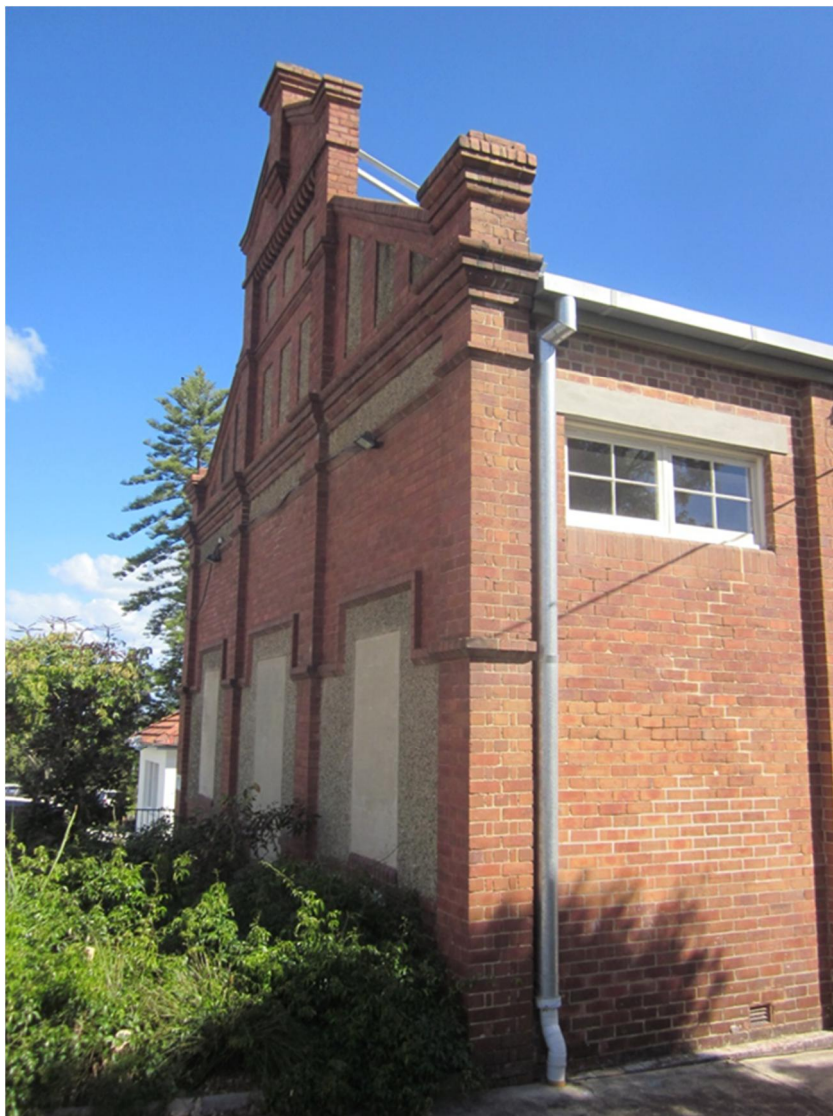
Figure 18. Eastern facade, showing new rainwater goods.
