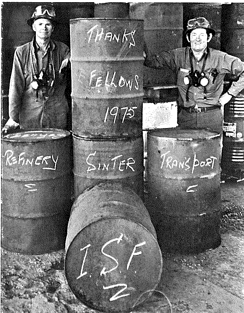
At around $10 each, the four hundred 44-gallon drums needed to store catalyst from the various units at D Acid Plant could have represented a sizable cost to the department except for the co-operation of other sections of the Works who between them managed to supply enough to fill the bill. The picture spells out the gratitude for their assistance. At left is, Shift Foreman, Joe McDougall and, at right, Day Foreman, Jack Raw.
