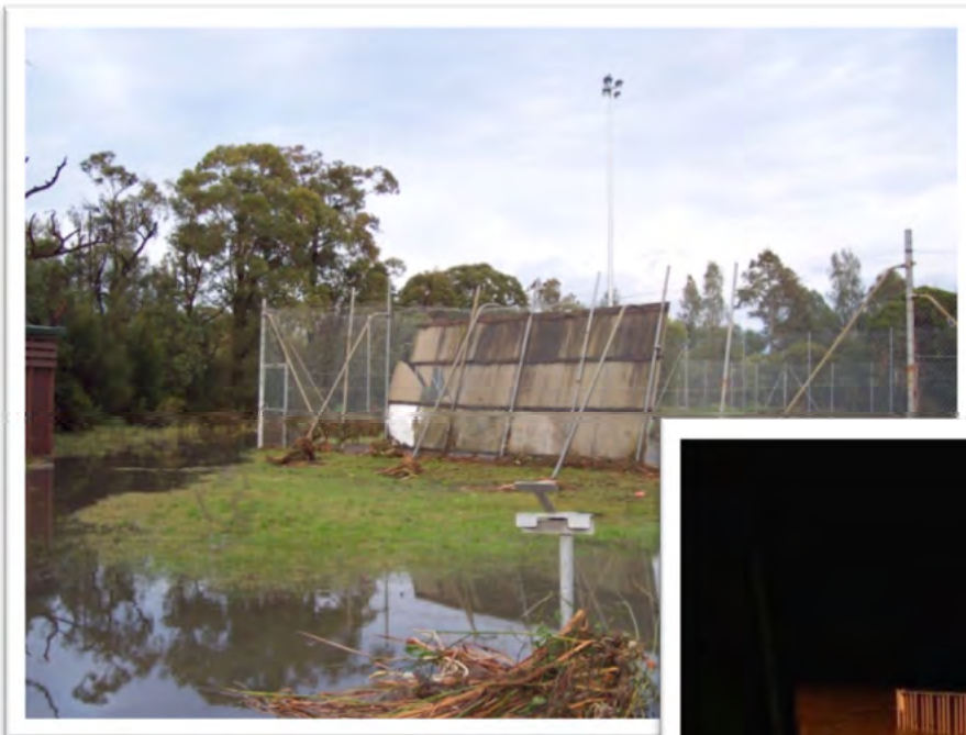
June 2007: Debris at Charles Street tennis courts
