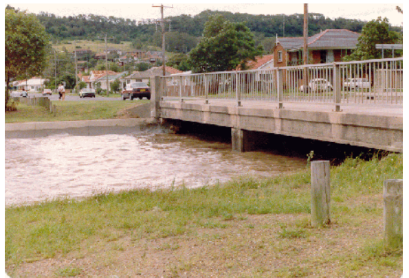
Floodphoto 6: The Esplanade Bridge - 4 Feb 1990
