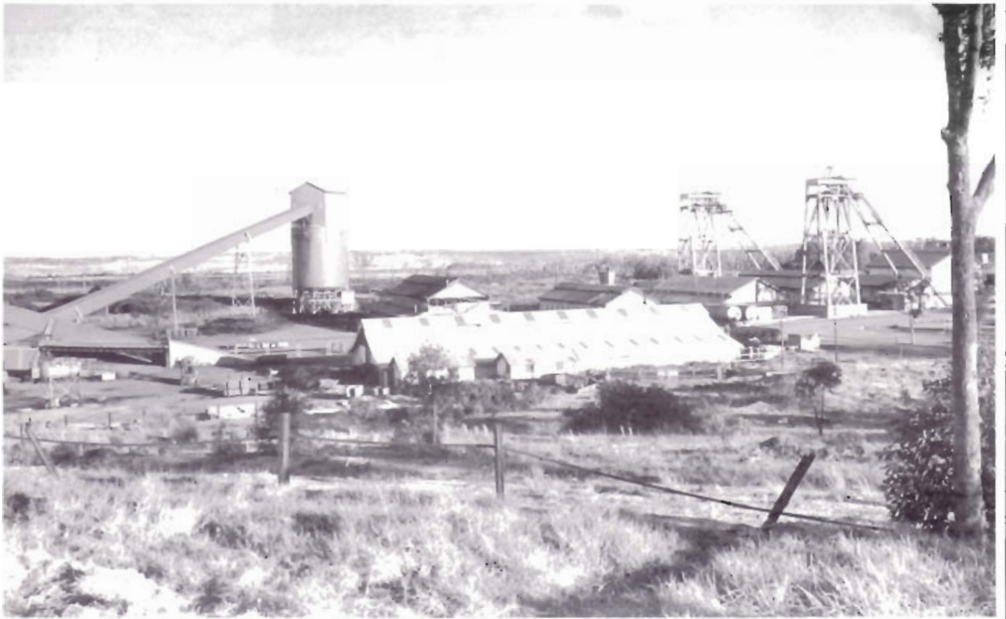
Top: 1969 - Looking south at storage bin and headframes with bulk store in foreground. Bottom left: 1980 - Surface layout.
