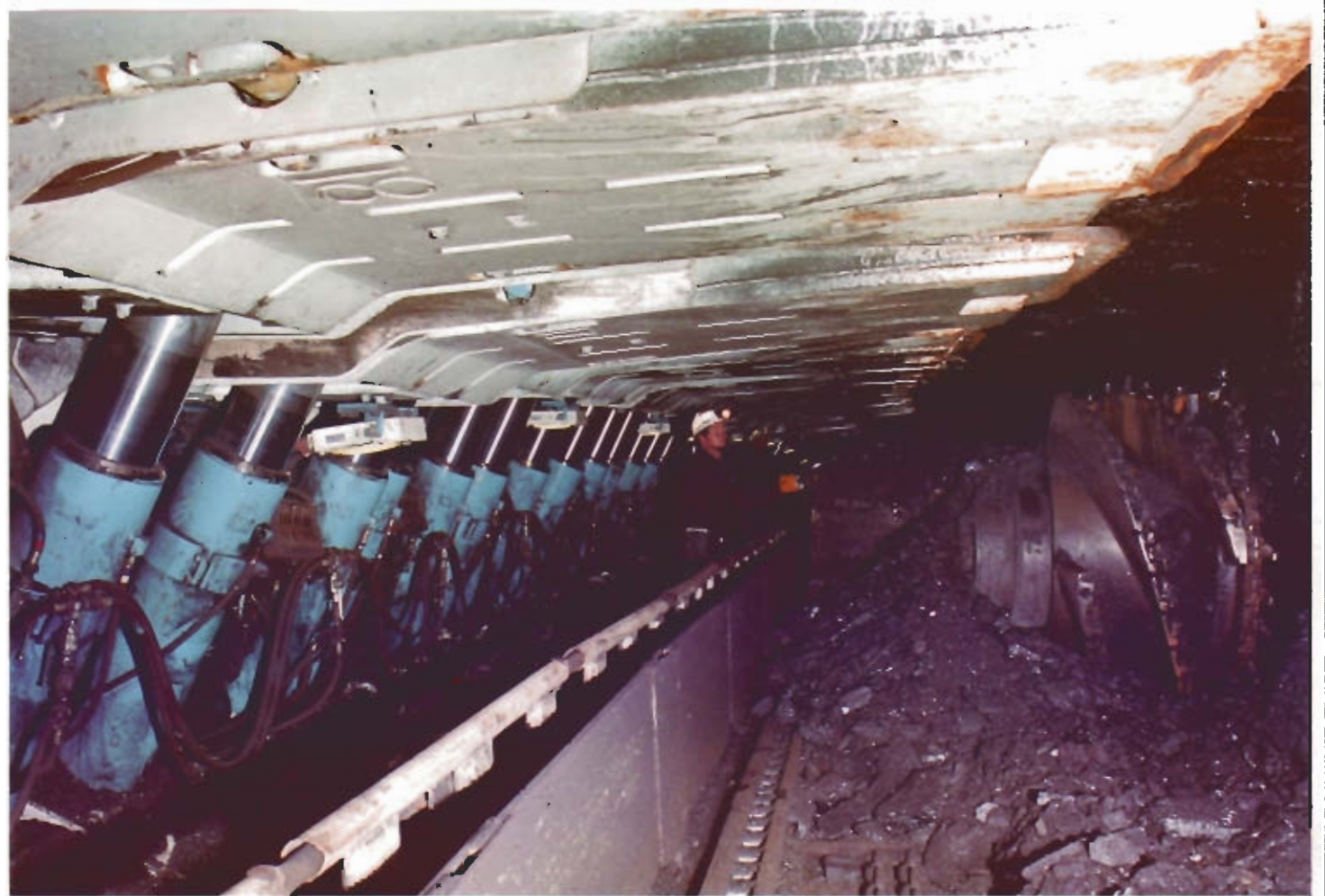
Longwall operation at John Darling Colliery.
