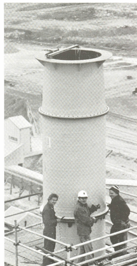
Rigger, Dave Oughton, L/H Boilermaker, John Neilson, and Rigger, Keith Wells, from contractors A. B. Rea, attaching stack extension after it was positioned by the helicopter.
