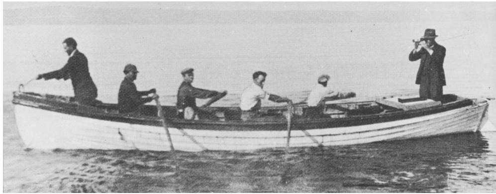
Exhibit 1 Whaleboats such as that shown above were being used for surveying Lake Mac from about 1827. Also used in: Fryer, John (Ed.), Surveying the Hunter, etc. , Institute of Surveyors (Hunter-Manning Group), 1980; where at p. 42 it is described as: "Sounding, as practiced from early times right up to the 1960s. The surveyor (right) holds the sextant and the man at the bow takes depth readings by means of a lead-weighted line."
