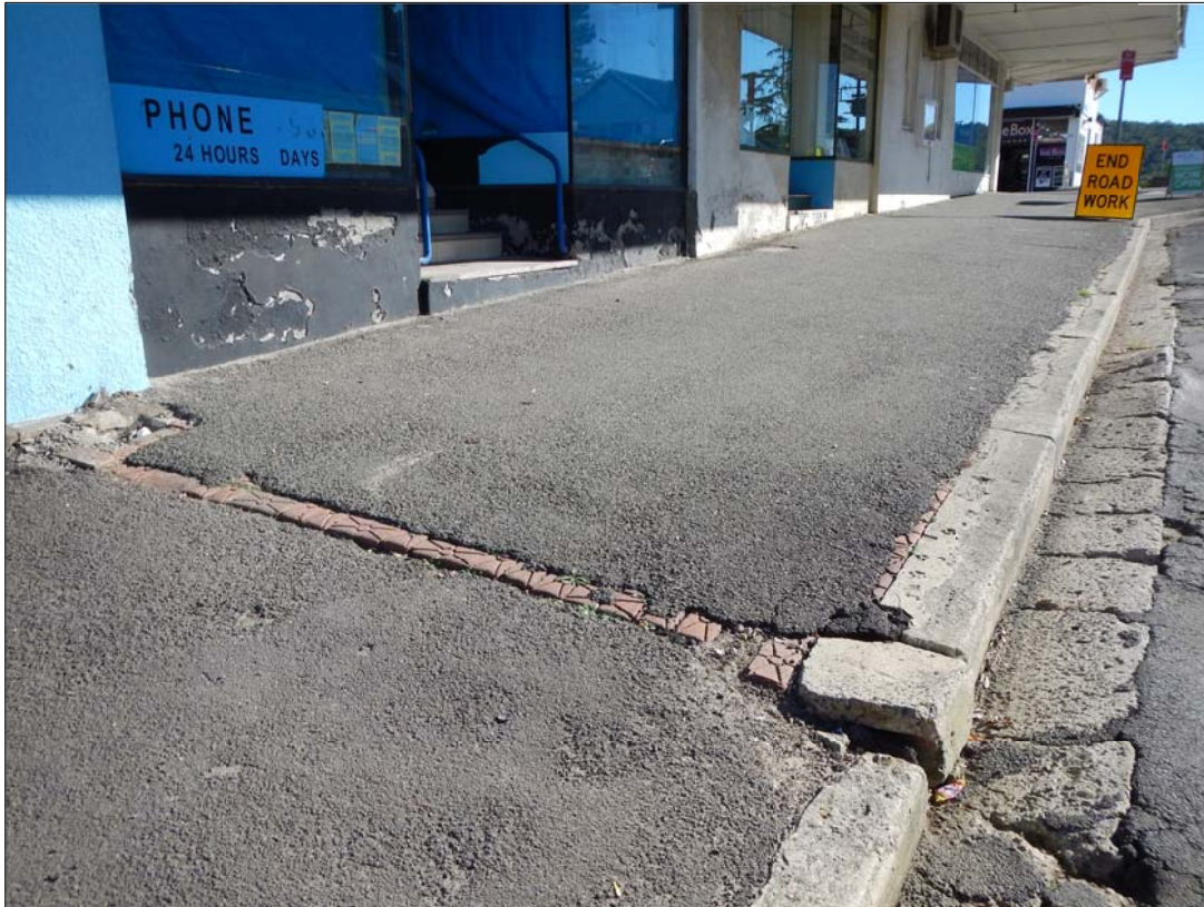
PLATE 3.1 View to north along west side of Withers Street to Carrington Street Corner showing 1930s pavers beneath asphalt footpath surface
