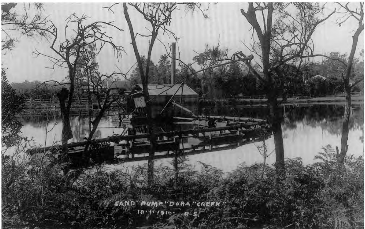
Photo below, an early form of dredging, a sand pump on the creek in 1910.
