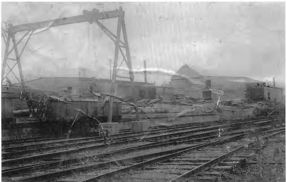
The railway side of Mullard's 'Top Mill' in Dora Street, Morisset. Finished timber was loaded directly onto the railway wagons. On the right is the chimney of the huge boiler, which provided steam energy for the machines in the mill. 'Darkie' the horse waits patiently near a loaded wagon. Photo Mary Barnes.
