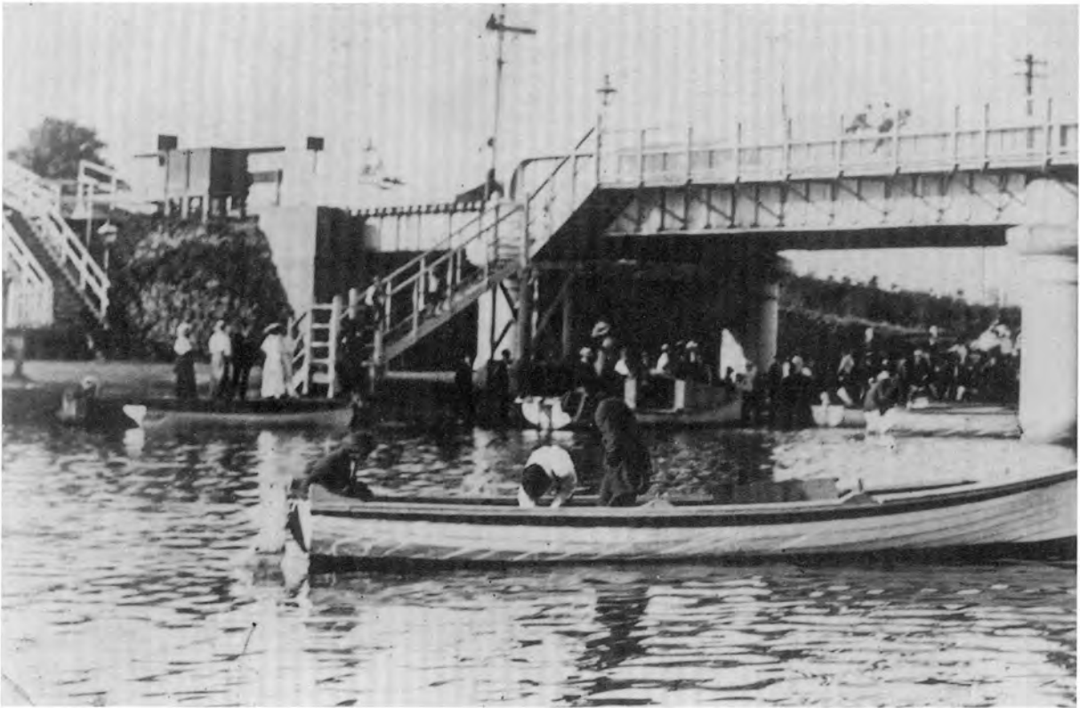
The opening of Dora Creek Railway Bridge, August 15 1889 was a great cause for excitement and celebrations. The bridge consisted of seven 60ft-plate iron spans.
